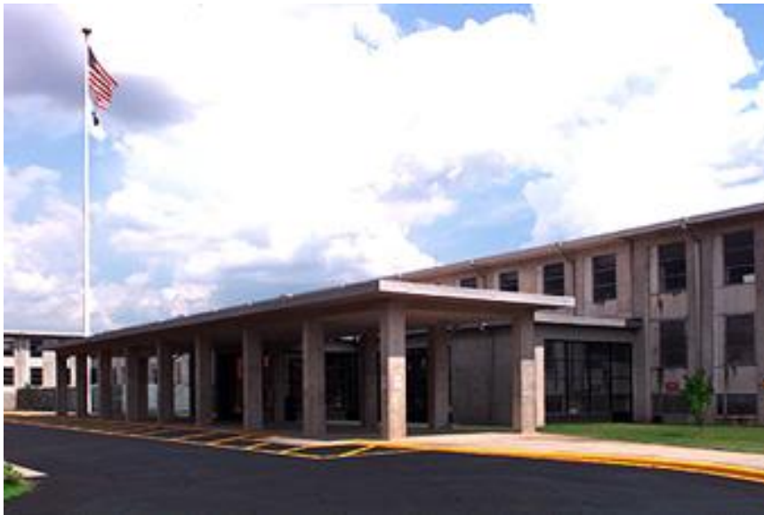
Savannah River Site
